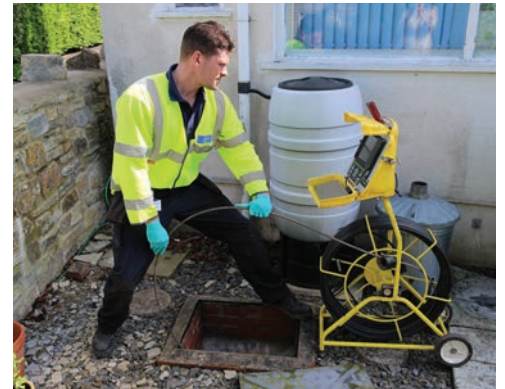
Carrying out a CCTV survey
